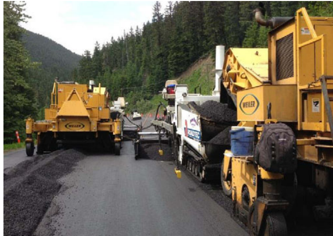
Photograph of paving work through Manning Park.
