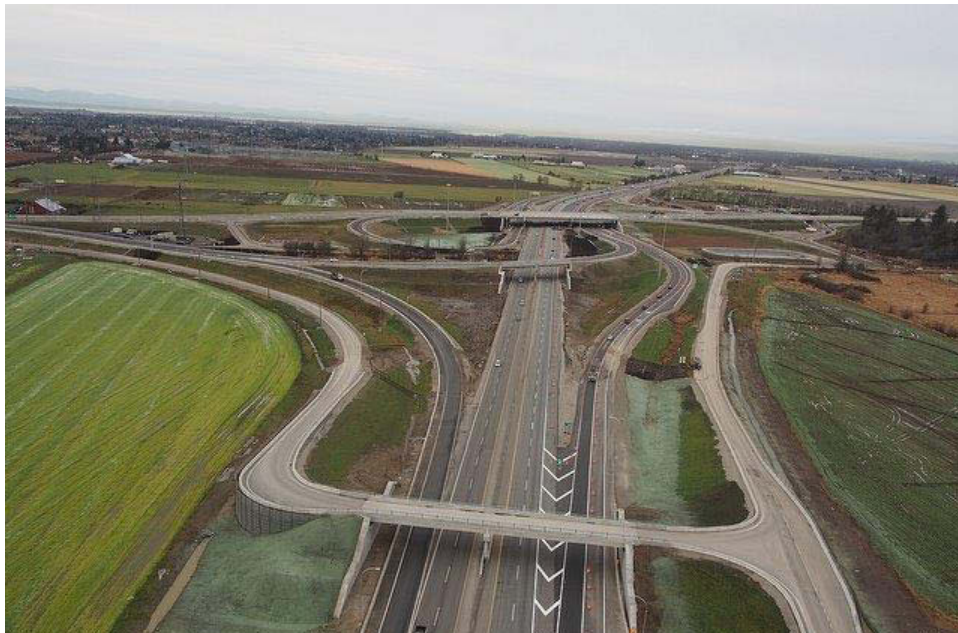
An aerial view of the Highway 99 Interchange on the new SFPR, with an agricultural overpass in the foreground.
