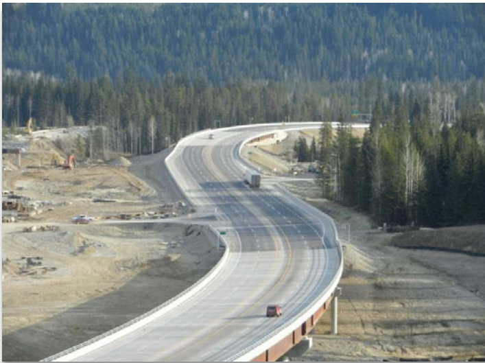
Aerial view of the new four-lane Donald Bridge, which opened to traffic in November 2012.
