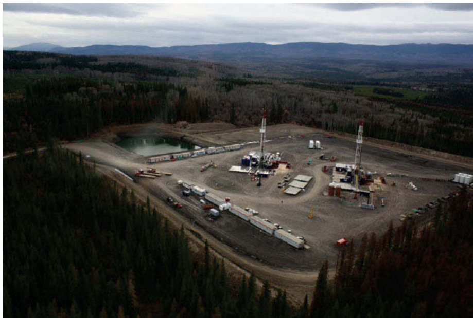
Talisman natural gas drilling rig near Fort Saint John, northeast B.C.
