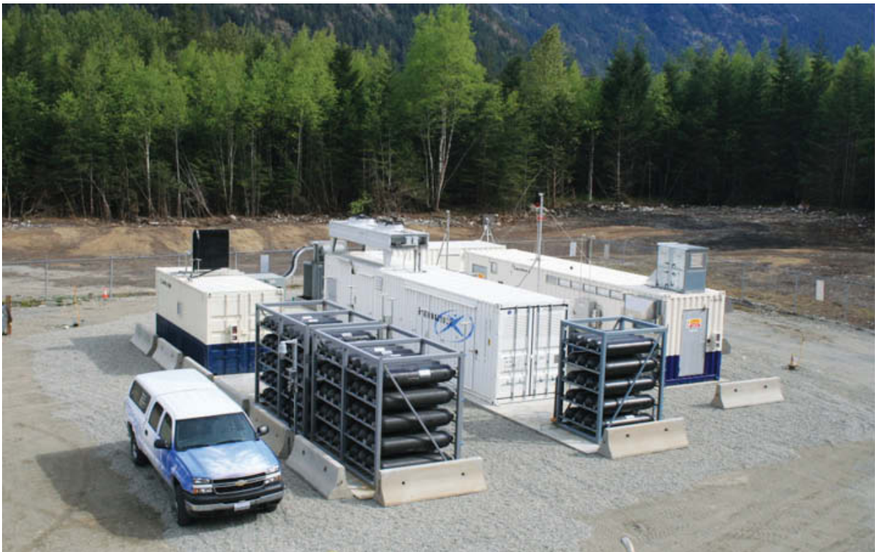
In Bella Coola, B.C., the Hydrogen-Assisted Renewable Power (HARP) project uses clean, green hydrogen and fuel cell technology to help power this remote community. Located approximately 400 kilometres north of Vancouver, Bella Coola is not connected to BC Hydro's provincial electricity grid.
