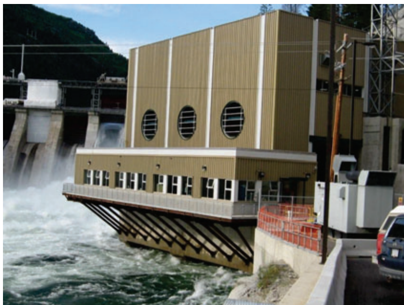
The 120 megawatt Brilliant expansion powerhouse is an addition to the 145 megawatt hydroelectric Brilliant dam on the Kootenay River near Castlegar, B.C.
