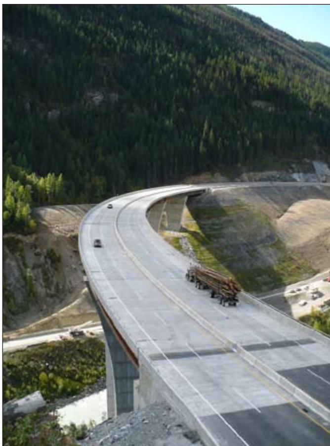
Traffic using the new Park Bridge
