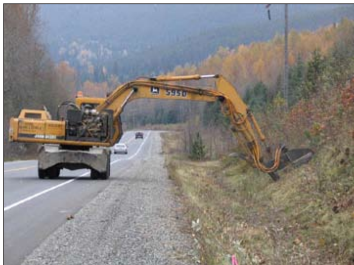
Highway shoulder maintenance — brush cutting
