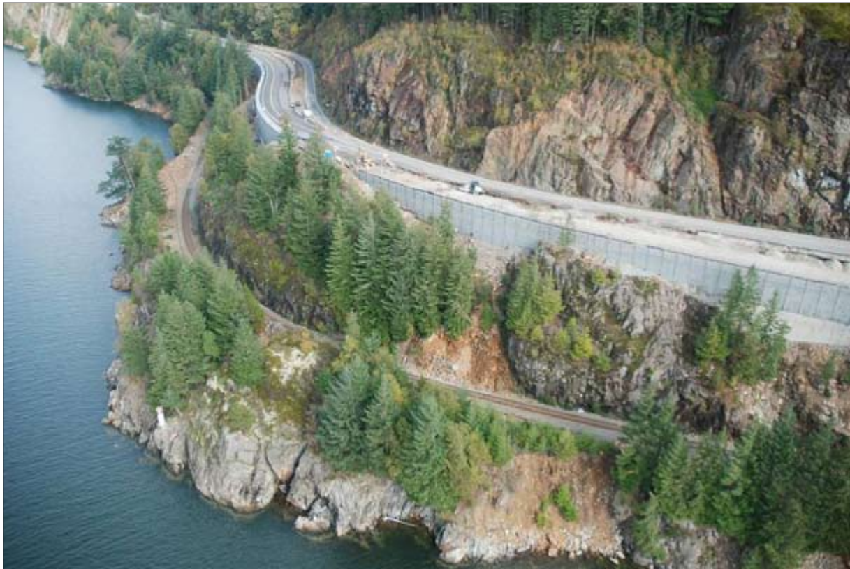
Mechanically stabilized earth walls to widen highway north of Lions Bay.
