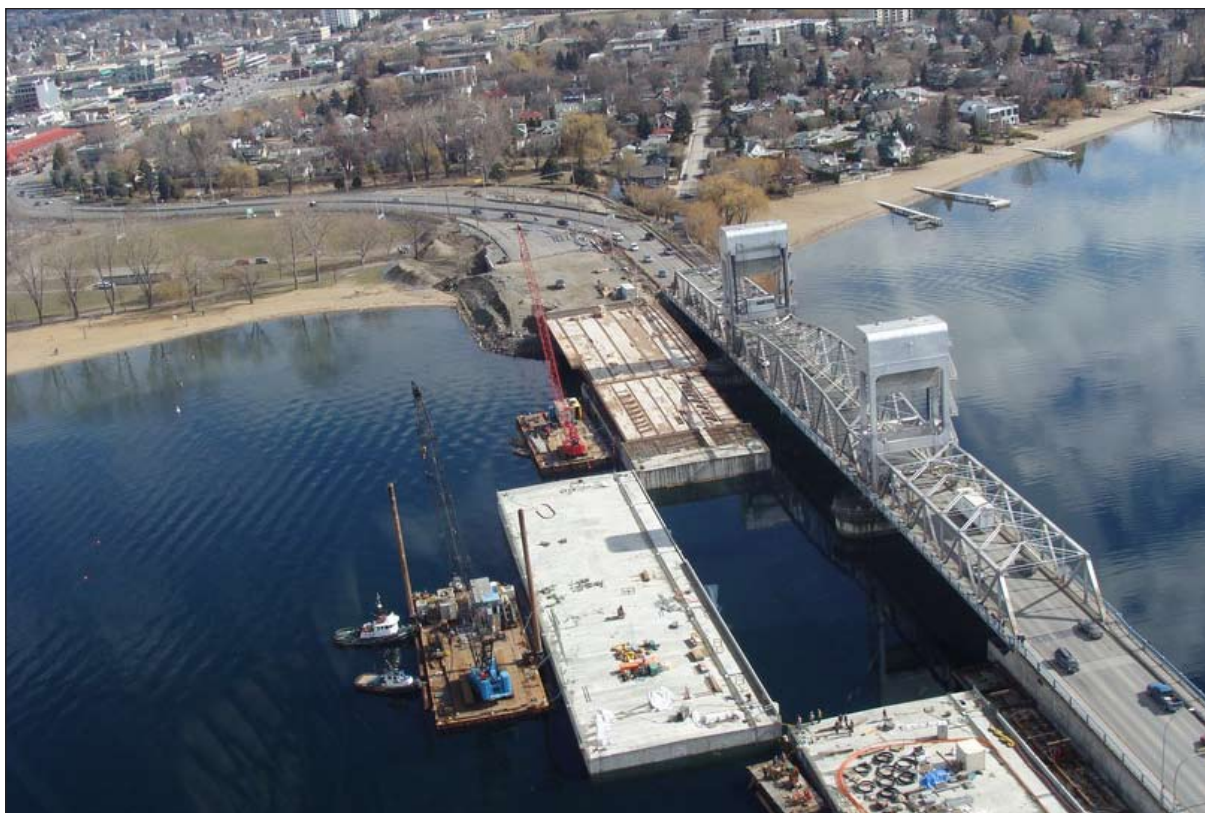
Installing the final pontoon section of the bridge.
