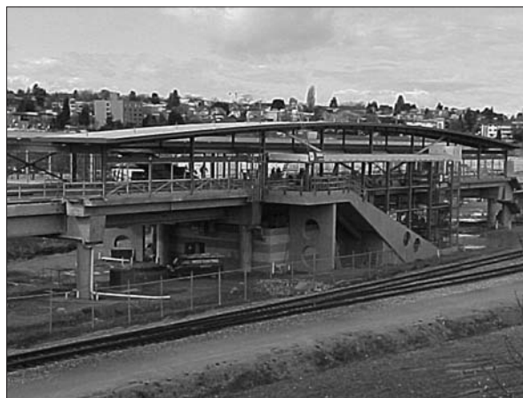
Vancouver Community College Station
