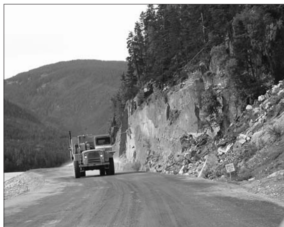
Lava Lake Construction — Nisga'a Highway
