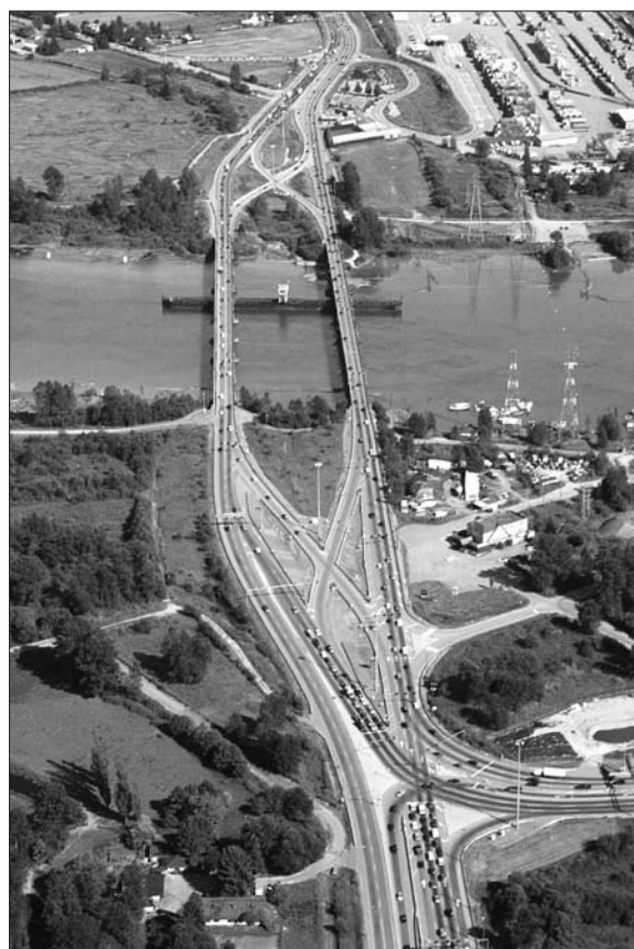
Pitt River Bridge
