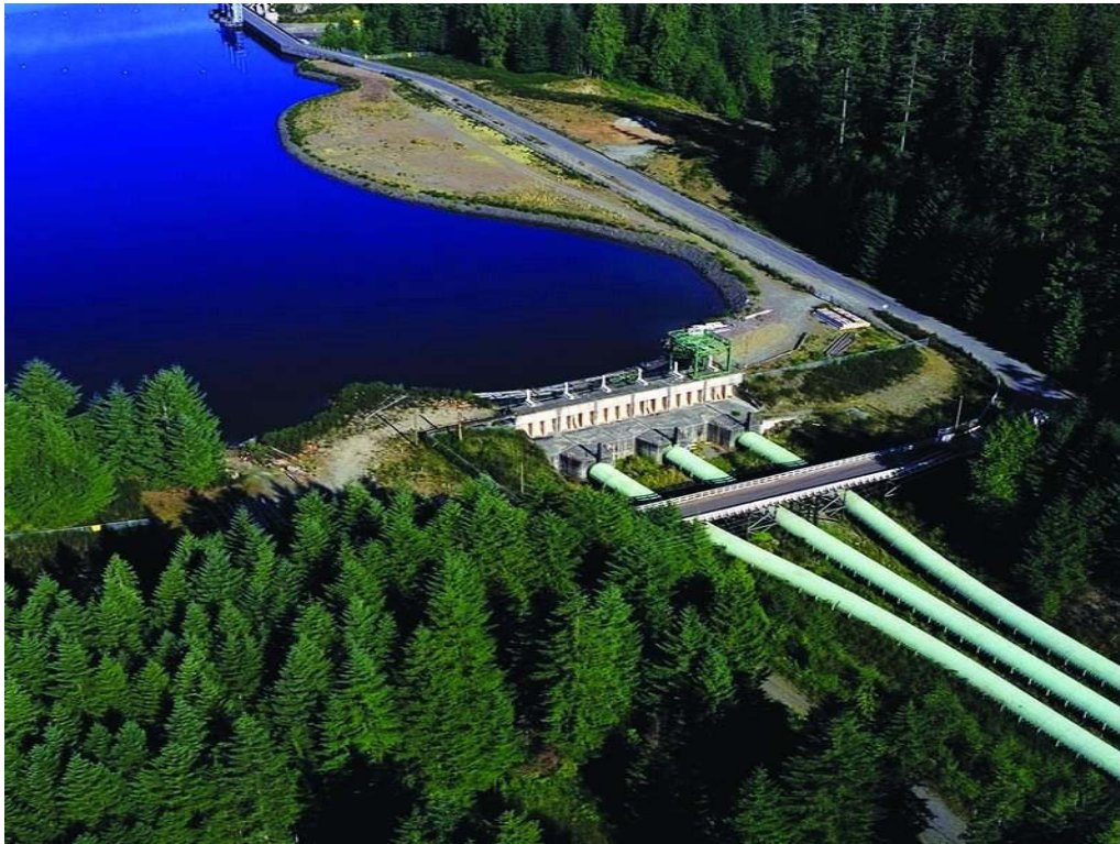
Photo: Courtesy BC Hydro
