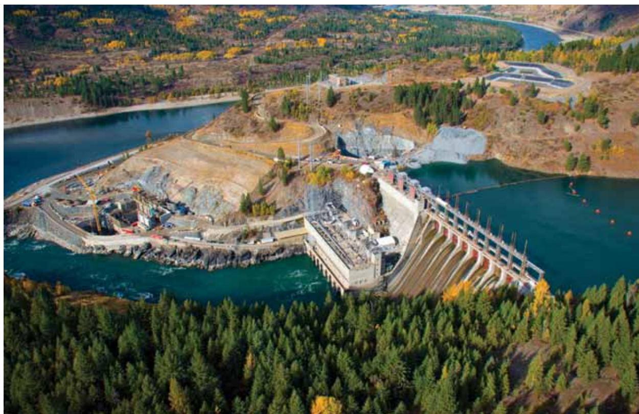
Aerial view of the Waneta Expansion Project, Fall 2012
