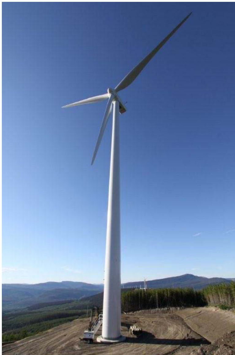
Dokie Ridge wind-powered electricity generating turbine located near Chetwynd, British Columbia.
