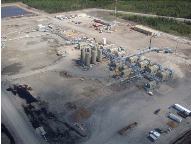
A multi-well pad site used for shale gas production in Northeast B.C.
