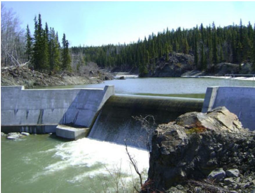
This hydroelectric dam near Atlin, B.C. reduces the community's reliance on diesel power.
