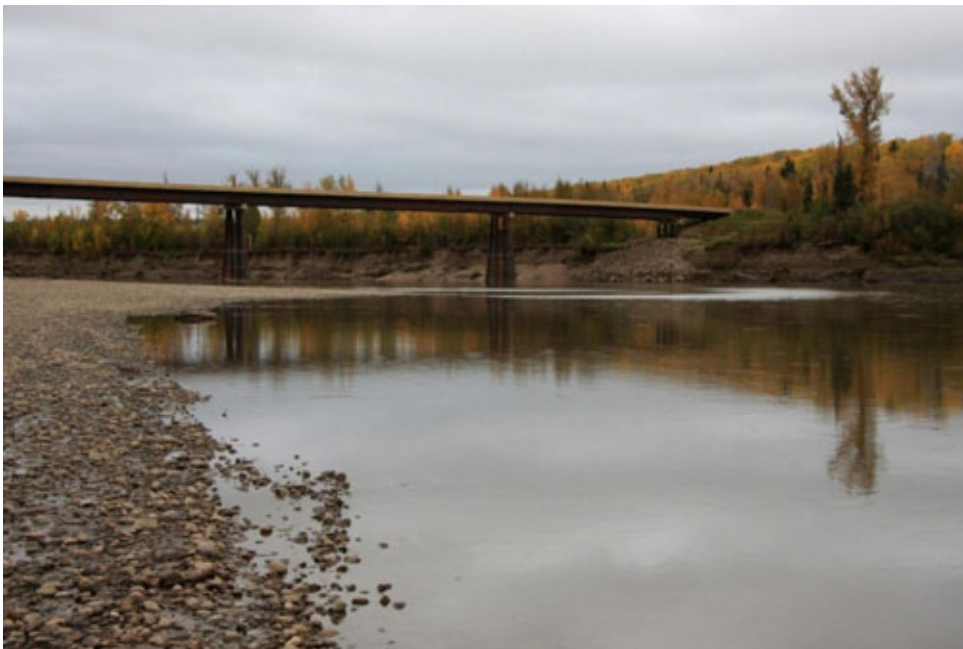
Sierra Yoyo Desan Resource Road, Northeast B.C.
