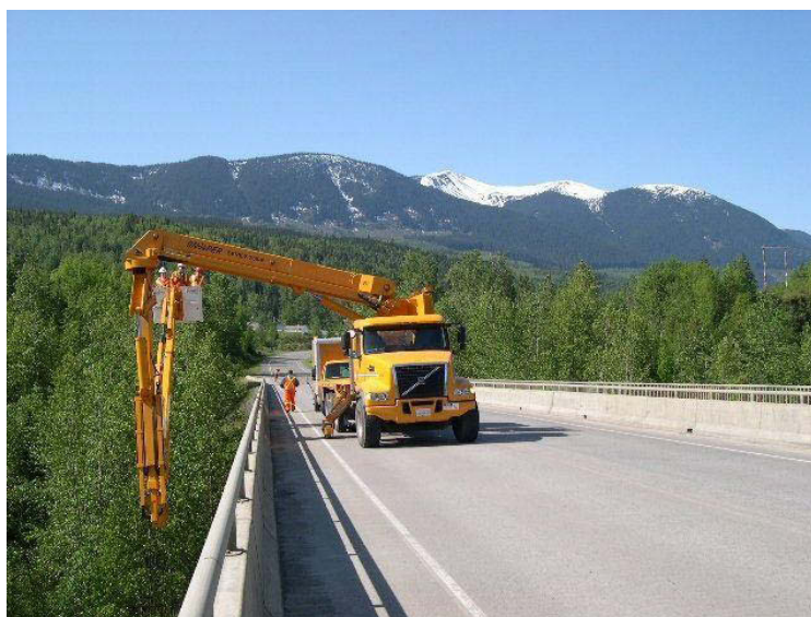
Bridge inspections with a Snoop truck.
