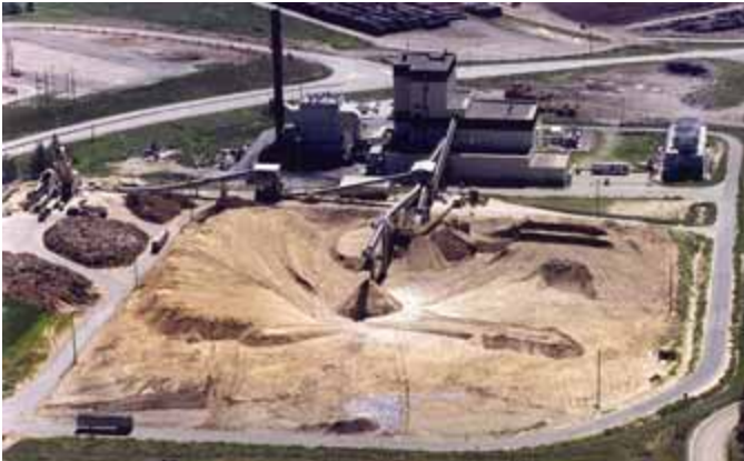
Wood residue power plant in Williams Lake, B.C.
