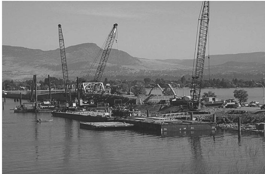
William R. Bennett Bridge construction site
