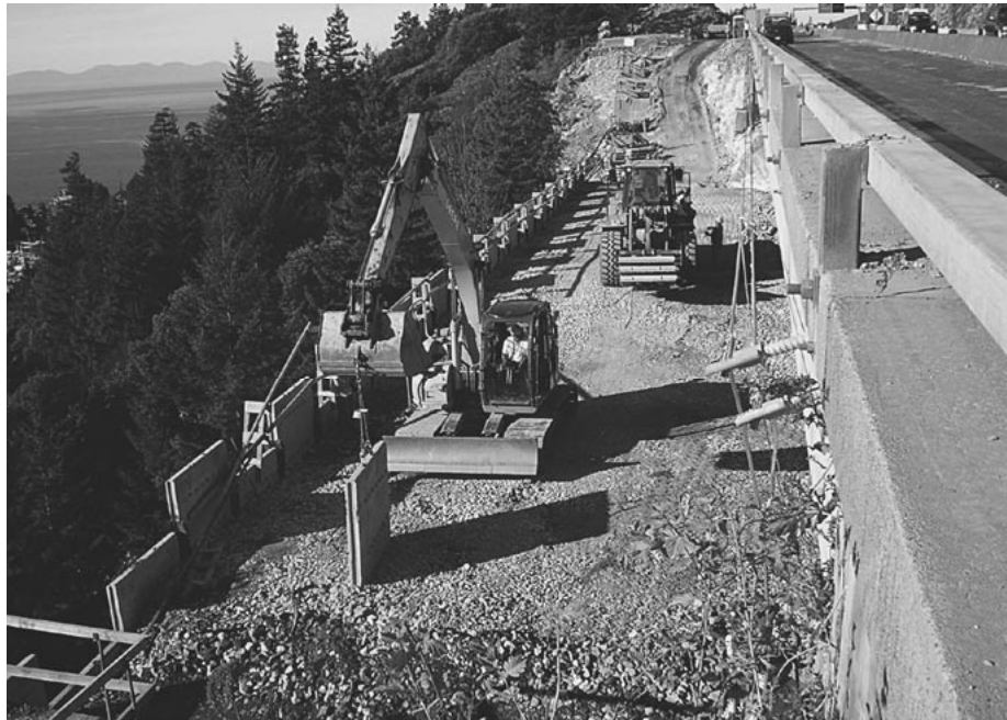
Sea-to-Sky Highway Improvement Project: Newly completed section through Furry Creek
