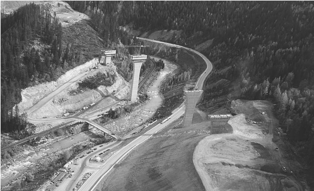
Kicking Horse Canyon – Park Bridge pier
