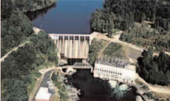
Ruskin Generating Station is located on the Stave River near its confluence with the Fraser River. The 105.6 megawatt powerhouse contains three generation units. A dam safety improvements project, planned for completion in 2009, will mitigate earthquake risk and protect public safety.
