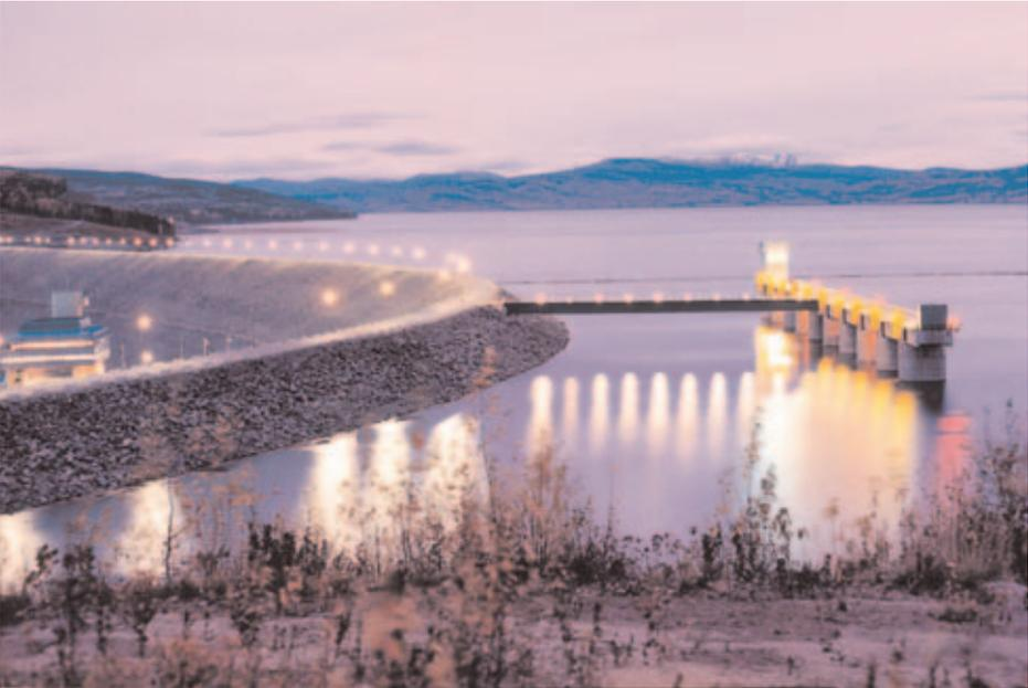
Built in September 1968, the WAC Bennett Dam is among the world's largest earthfill dams. Together with the 10-unit GM Shrum (GMS) Generating Station it comprises the Portage Mountain Project. A stator upgrade project, planned for completion in 2012, will reduce the number of forced outages and related financial impacts.
