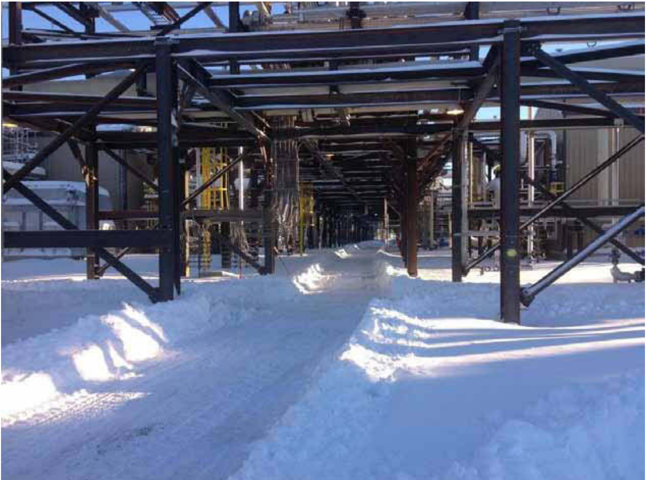
Cabin gas plant project
