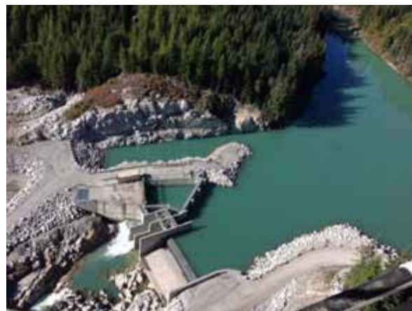
Upper Harrison Hydroelectric Project – Intake and headpond.
