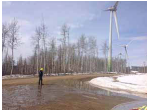
Bear Mountain Wind Park Project – Compliance Inspection
