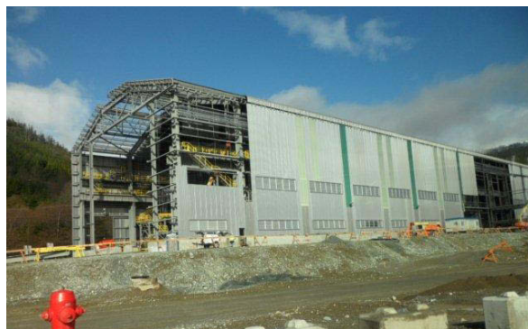
Structure for new pot lines at the Rio Tinto Alcan smelter modernization project in Kitimat, BC.
