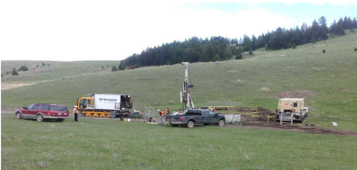
Geotechnical drilling at proposed Ajax Mine Site
