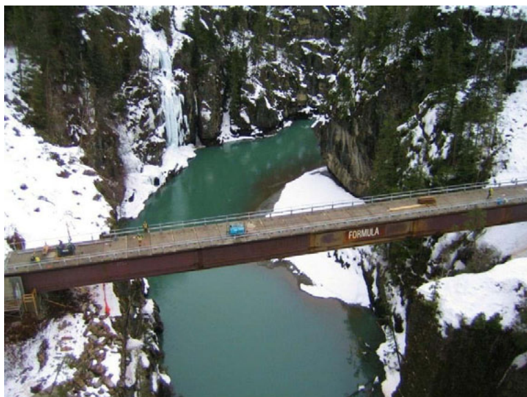
Compliance site inspection for the McLymont Creek Project over the Iskut River.
