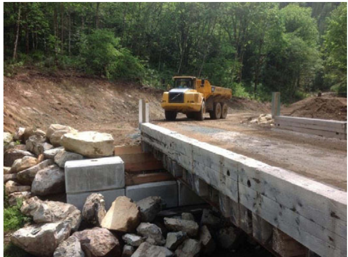
Construction on the access road for the Interior to Lower Mainland Transmission Project.
