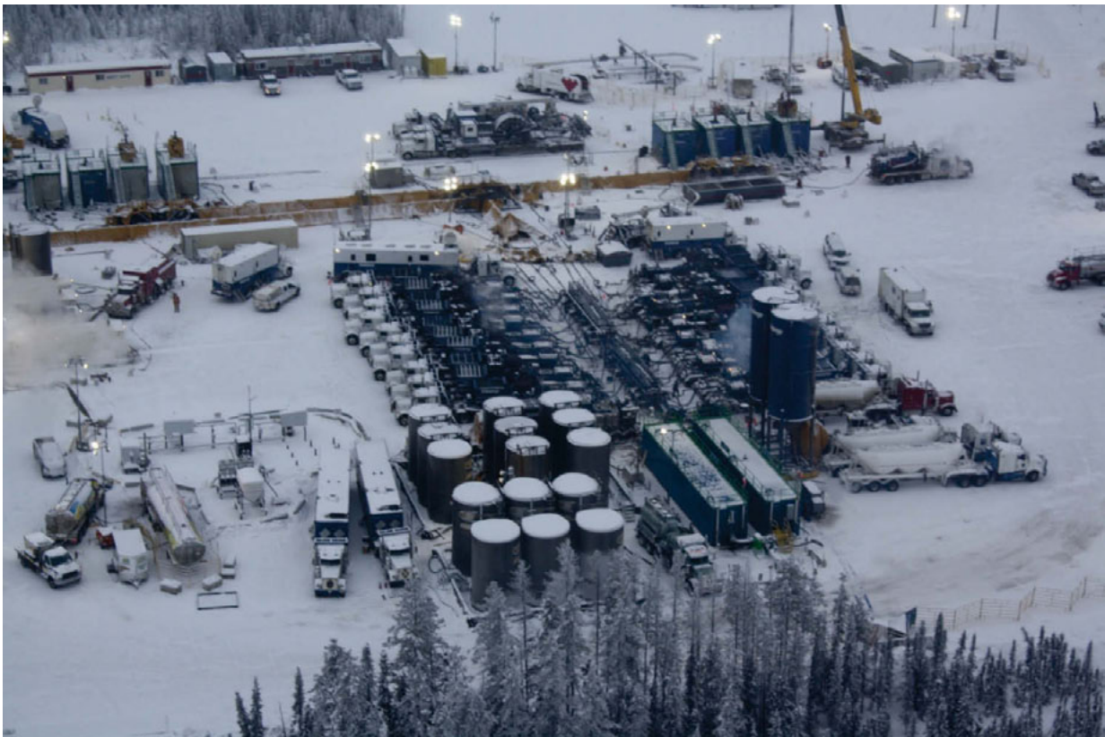
A site with multiple natural gas wells in Northeast B.C.
