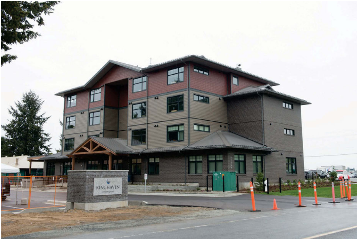
The George Schmidt Centre in Abbotsford provides 30 units of supportive housing and is operated by the Kinghaven Peardonville House Society. This facility recently achieved the Leadership in Energy and Environmental Design (LEED) Gold certification.
