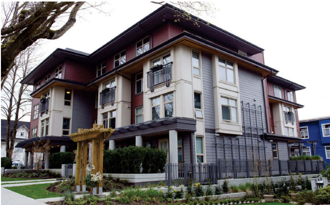
Linden Tree Place in Vancouver provides 30 affordable rental apartments for seniors and persons with disabilities and is operated by Kits Neighbourhood House. The four-storey wood-frame building includes 10 wheelchair-accessible apartments designed for people with physical disabilities.
