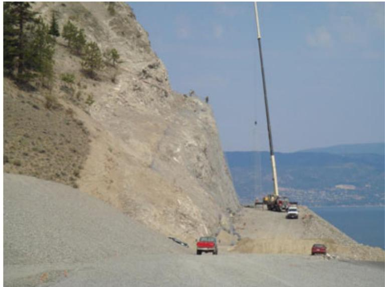
*Workers install mesh to keep rock off the travelled roadway as part of the Highway 97, Bentley Road to Okanagan Lake Park Project.*
