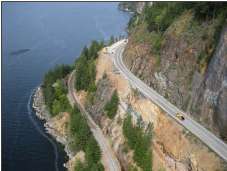
Sea-to-Sky Highway Improvement Project: Newly completed section through Furry Creek
